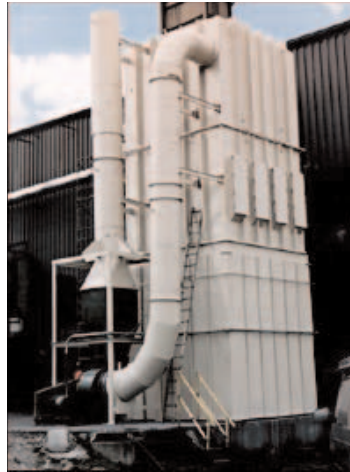
Pulse-jet Cleaning Collector (Photo Courtesy of C.P.E. Filters Inc)
