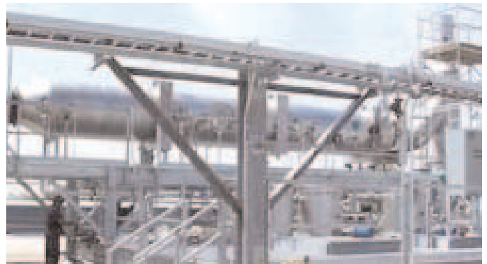
Wet Scrubber (Photo courtesy of Turbosonic Inc.)
